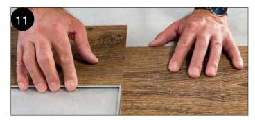
DISASSEMBLING THE SHORT SIDE Disassemble the row by sliding apart the planks on the short side.
