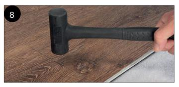
SECURING PLANKS As you go, don't forget to use a rubber mallet and tapping block on the short sides to secure the locking.
